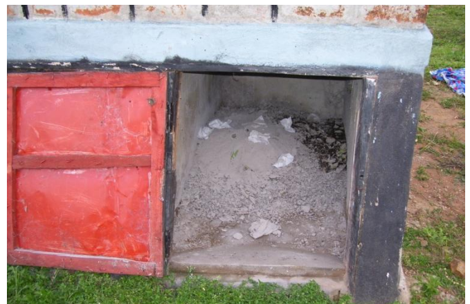
Fig. 7: Faeces collection chamber half way full (source: David Watako, GTZ-Kenya, July 2009)
