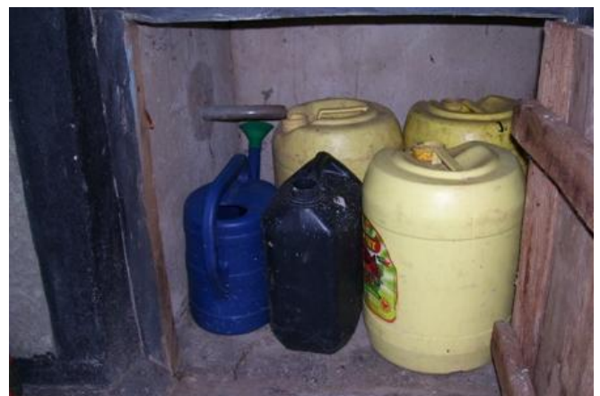
Fig. 8: Urine collection chamber with a number of urine containers/jerry cans (source: Moses Wakala, GTZ-Kenya, Jan. 2010)
