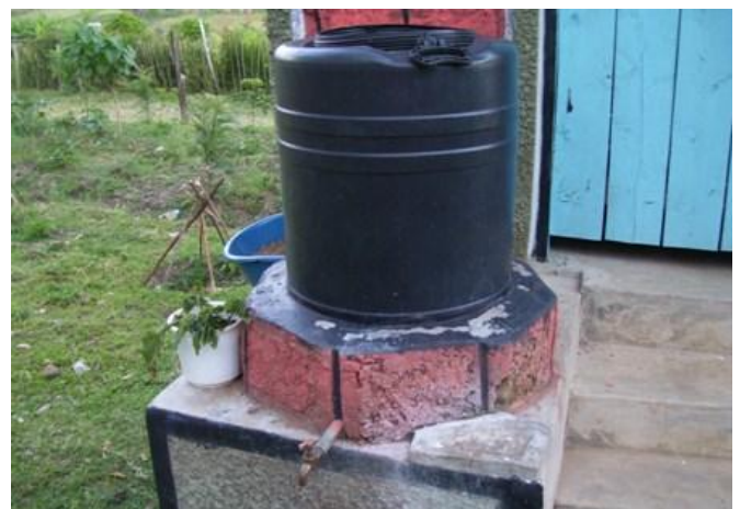
Fig. 6: Hand wash facility with 100 liter tank secured in concrete (source: Moses Wakala, GTZ-Kenya, Jan. 2010)
