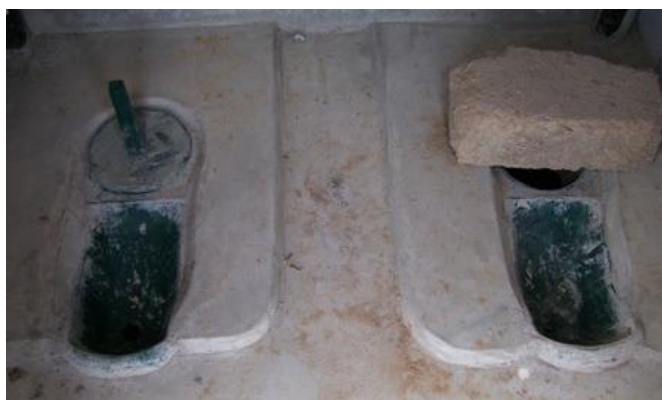
Fig. 10: Inside of a Urine diversion dehydration toilet (UDDT) using 2 single hole squatting pans near Wajir done by ALDEF (source Paul Mboya, GTZ-Kenya, June 2008)
