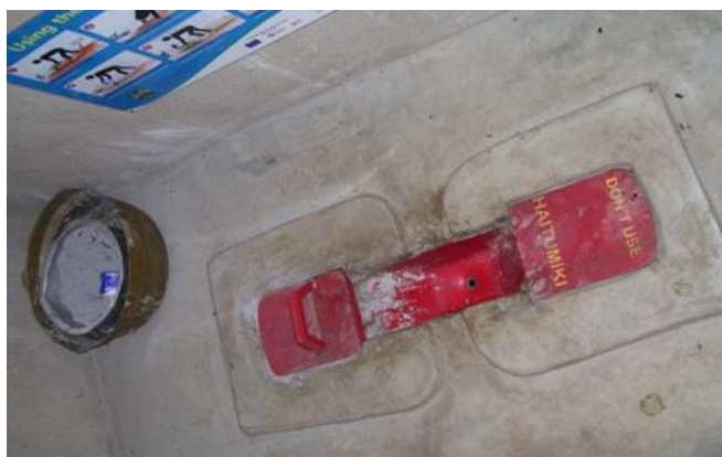
Fig. 9: Inside of a Urine diversion dehydration toilet (UDDT) with ash container, scoop and instruction posters
