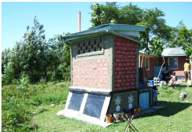
Fig. 5: Back view of household UDDT in Bungoma with faeces chambers and ventilation design (source Moses Wakala, GTZ-Kenya, Jan. 2010)
